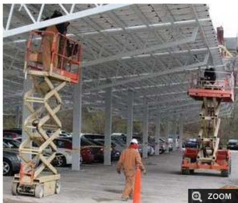
Workers install the final panels in the Cincinnati Zoo's new solar array. / The Enquirer/Ernest Coleman
